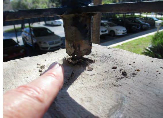
28 Level 2 Walkway Railing Corner Support Post Corroded Through Left Side of Building
