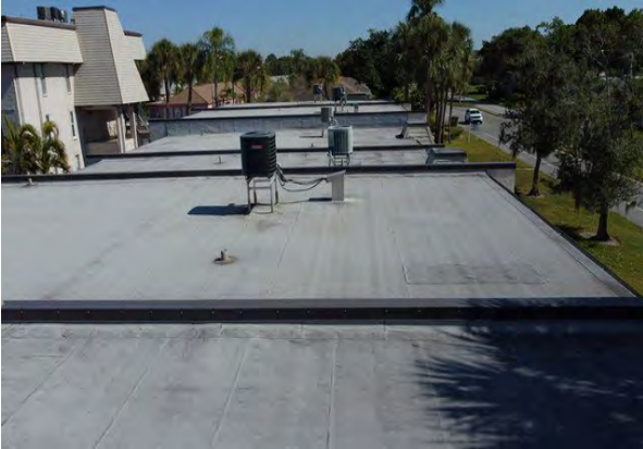
98 Building 8605 Roof Overview
