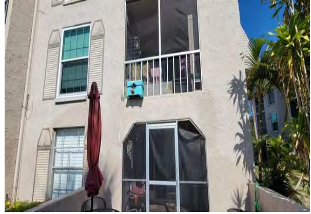
4 Left Rear Side of Building
