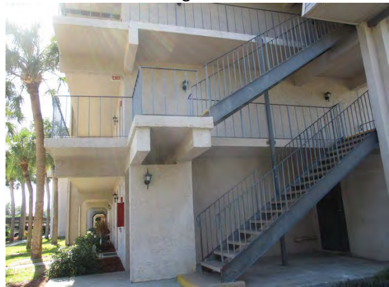
30 Right Side of Building 8693
