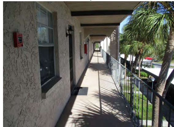
16 3rd Floor Walkway
