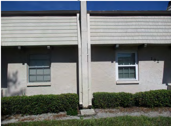
84 Front of Building 8605
