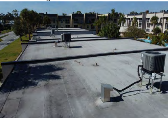
100 Building 8605 Roof Overview
