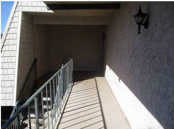
15 3rd Floor Walkway & Stairwell
