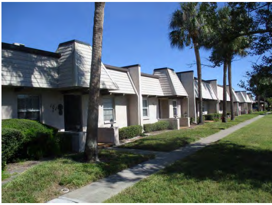
80 Front of Building 8605
