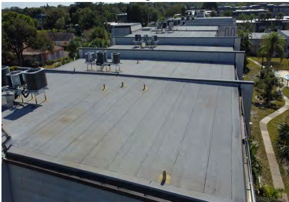
39 Roof Overview Building 8693
