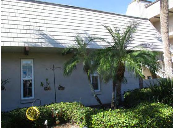
90 Right Side of Building 8605
