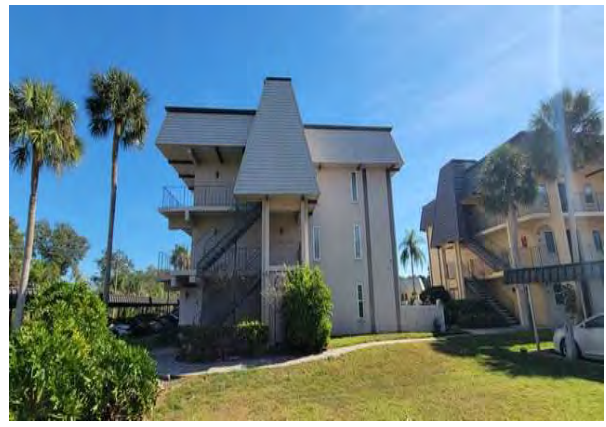
2 Right Side of Building
