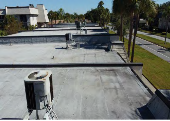
96 Building 8605 Roof Overview
