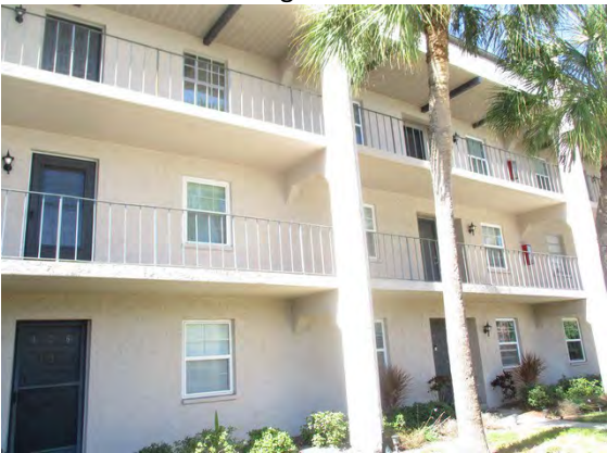
29 Front of Building 8693
