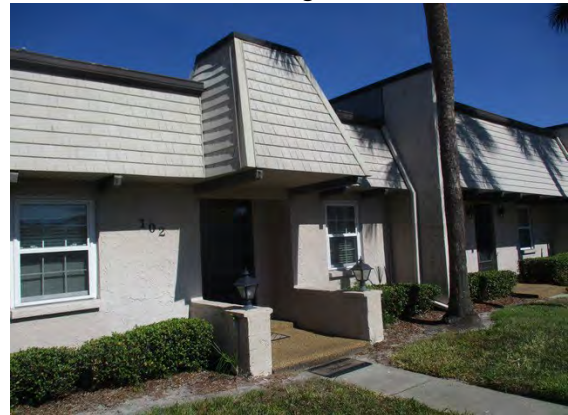
85 Front of Building 8605
