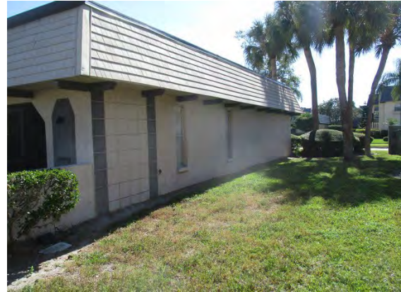
83 Left Side of Building 8605
