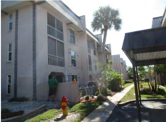
3 Rear of Building 8693
