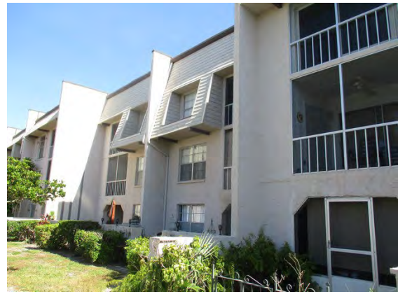
34 Rear of Building 8693
