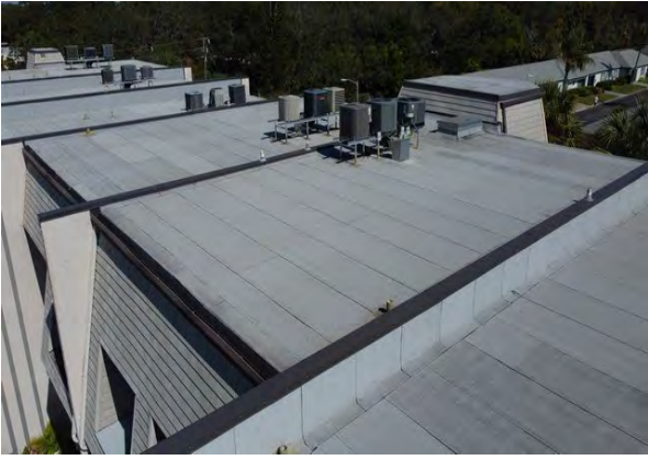
41 Roof Overview Building 8693
