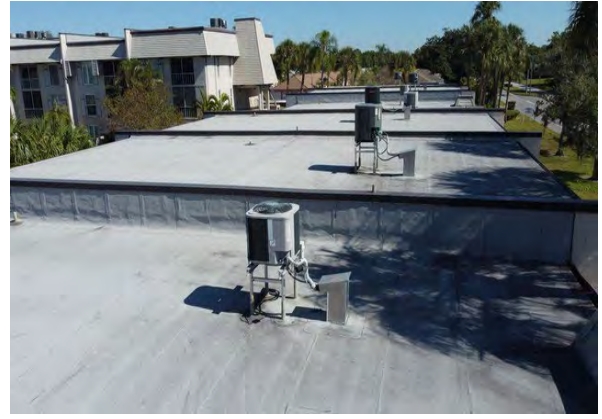
97 Building 8605 Roof Overview
