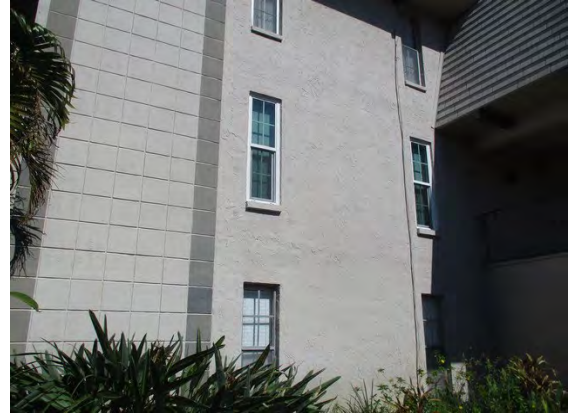
36 Left Side of Building 8963
