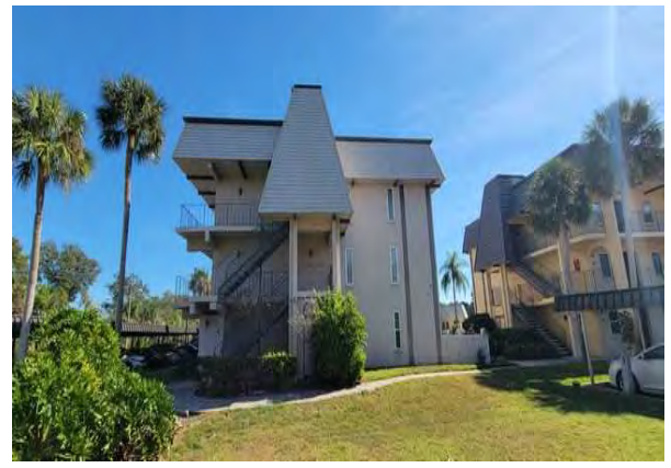
2 Right Side of Building
