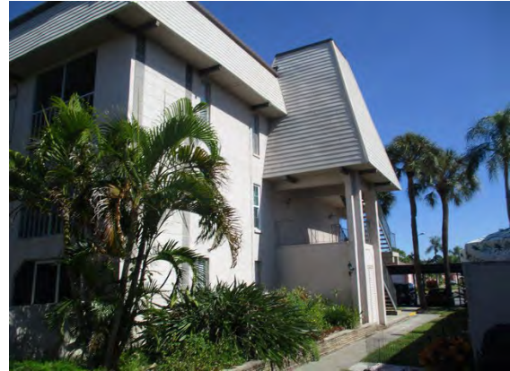
4 Left Side of Building 8693
