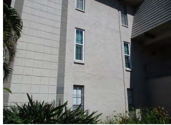
36 Left Side of Building 8963
