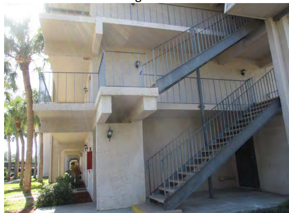
30 Right Side of Building 8693
