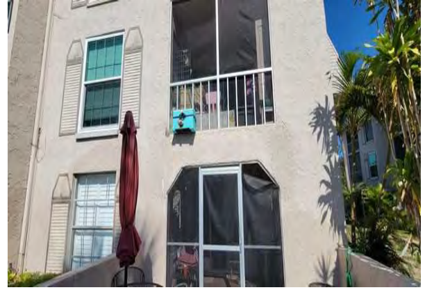
4 Left Rear Side of Building
