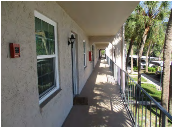
21 2nd Floor Walkway
