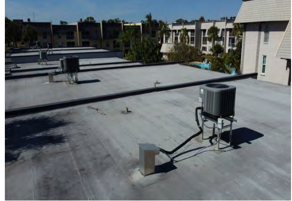
99 Building 8605 Roof Overview
