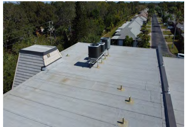
40 Roof Overview Building 8693
