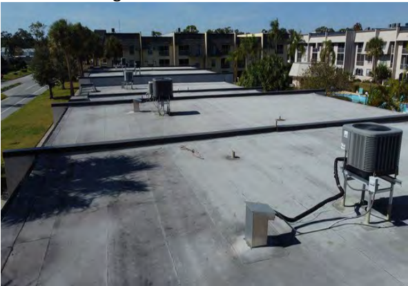
100 Building 8605 Roof Overview
