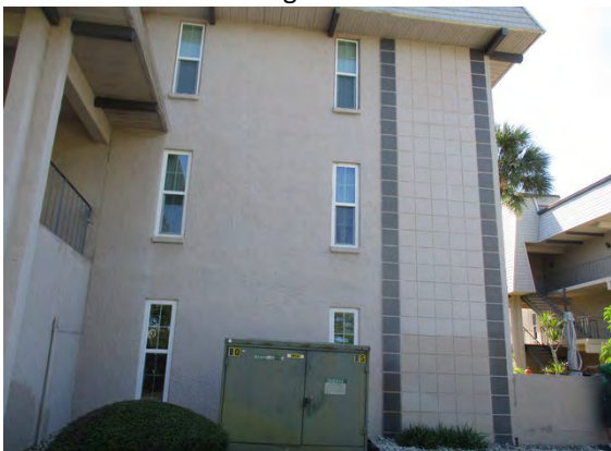
31 Right Side of Building 8693
