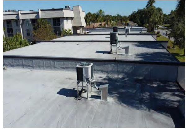
97 Building 8605 Roof Overview
