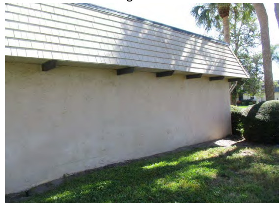
95 Left Side of Building 8605
