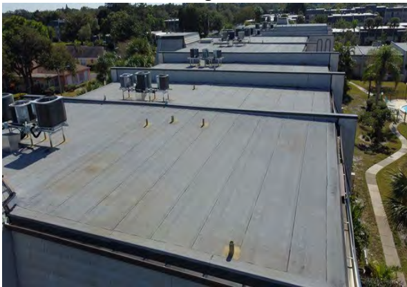
39 Roof Overview Building 8693
