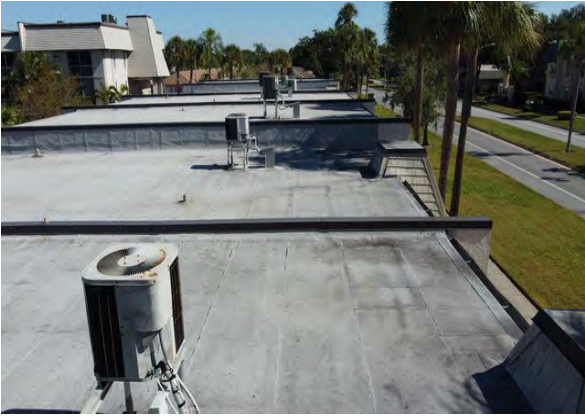
96 Building 8605 Roof Overview
