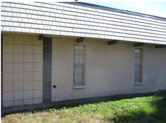
94 Left Side of Building 8605
