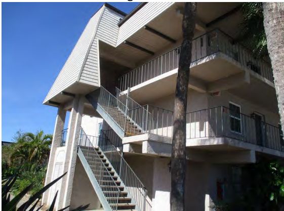
37 Left Side of Building 8963
