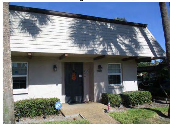
87 Front of Building 8605
