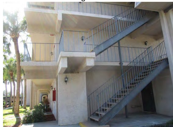
30 Right Side of Building 8693
