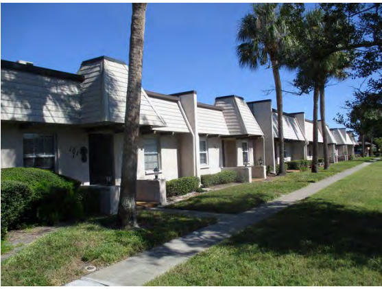
80 Front of Building 8605
