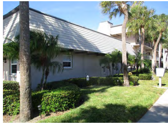
81 Right Side of Building 8605
