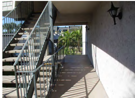
22 2nd Floor Walkway & Stairwell
