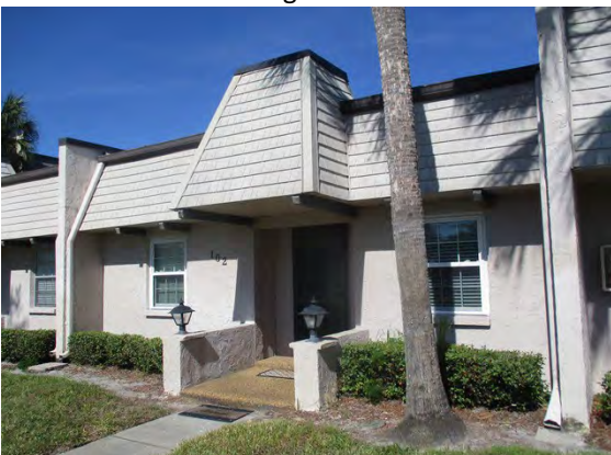
86 Front of Building 8605
