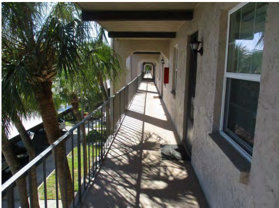
13 3rd Floor Walkway
