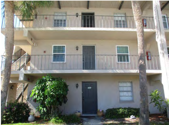
27 Front of Building 8693
