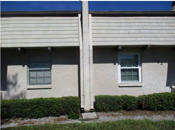
84 Front of Building 8605
