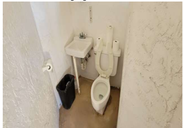
110 Pool Area Restroom
