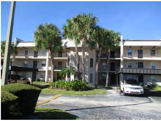
1 Front of Building 8693
