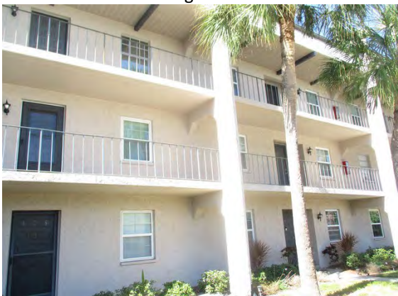
29 Front of Building 8693
