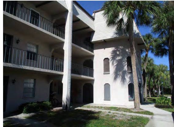
28 Front of Building 8693
