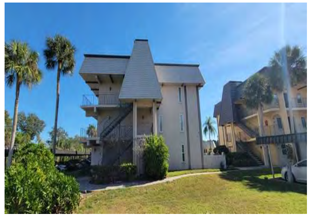
2 Right Side of Building
