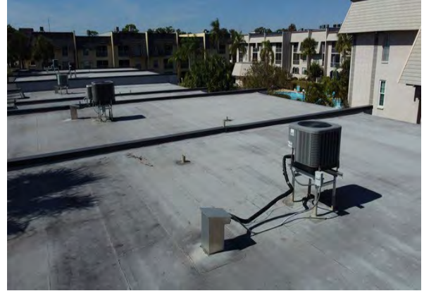
99 Building 8605 Roof Overview
