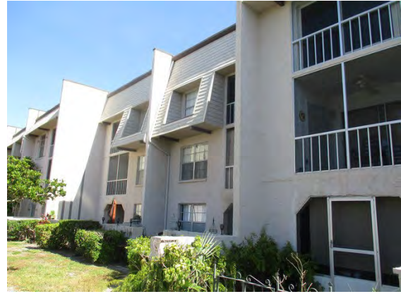
34 Rear of Building 8693
