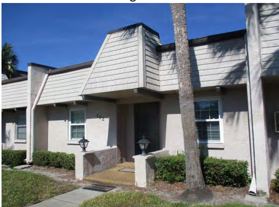
86 Front of Building 8605
