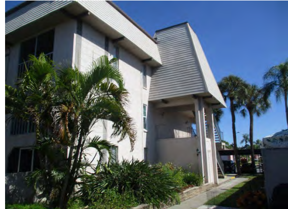
4 Left Side of Building 8693
