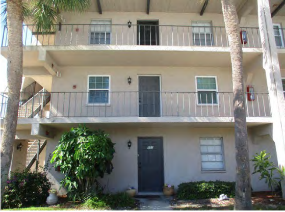
27 Front of Building 8693
