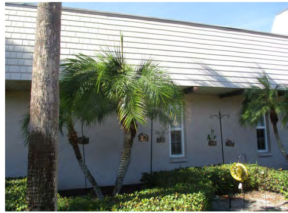
89 Right Side of Building 8605
