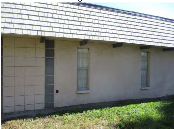
94 Left Side of Building 8605
