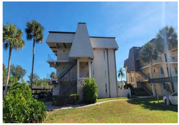
2 Right Side of Building
