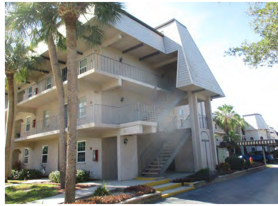
2 Right Side of Building 8693
