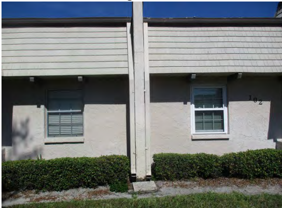
84 Front of Building 8605
