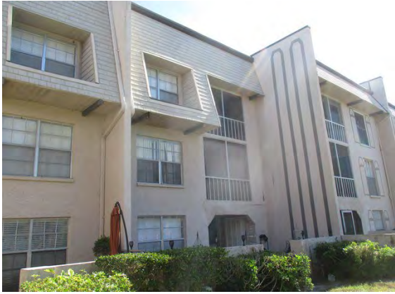
33 Rear of Building 8693
