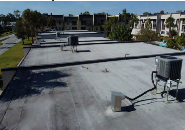
100 Building 8605 Roof Overview
