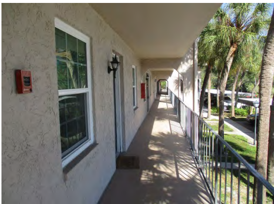
21 2nd Floor Walkway
