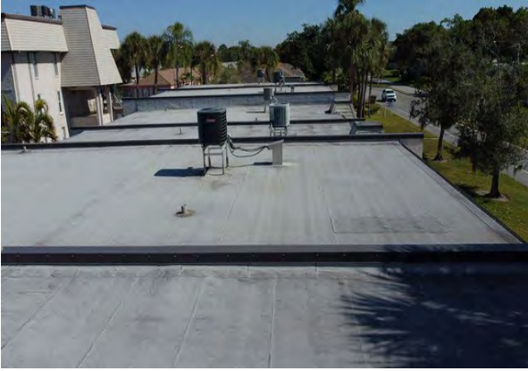
98 Building 8605 Roof Overview
