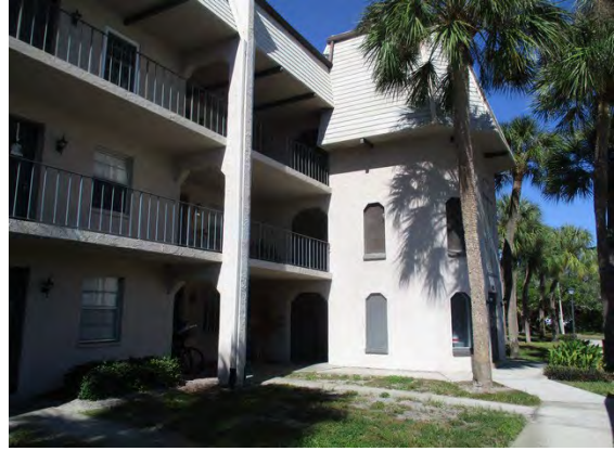
28 Front of Building 8693
