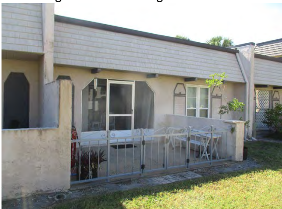
92 Rear of Building 8605
