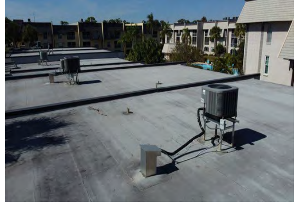
99 Building 8605 Roof Overview
