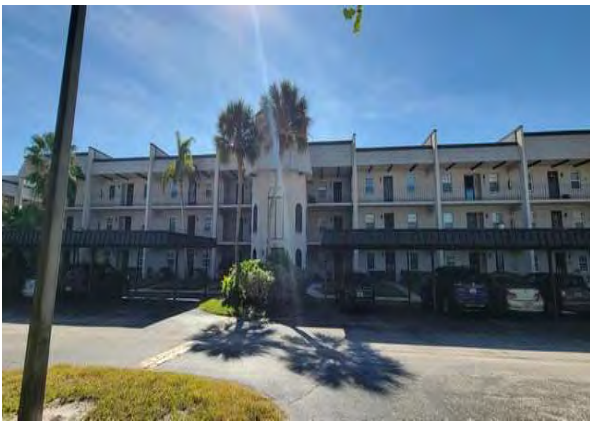
1 Front of Building
