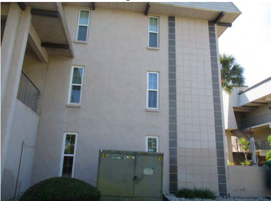
31 Right Side of Building 8693
