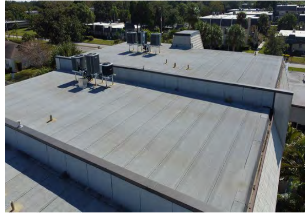
42 Roof Overview Building 8693
