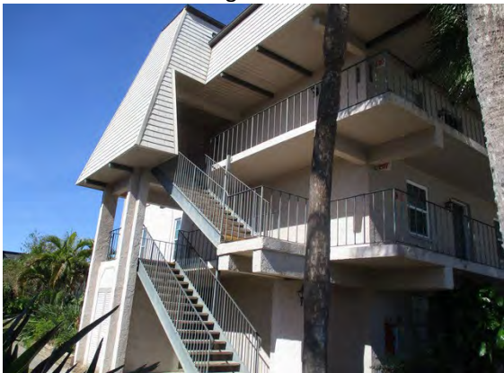
37 Left Side of Building 8963
