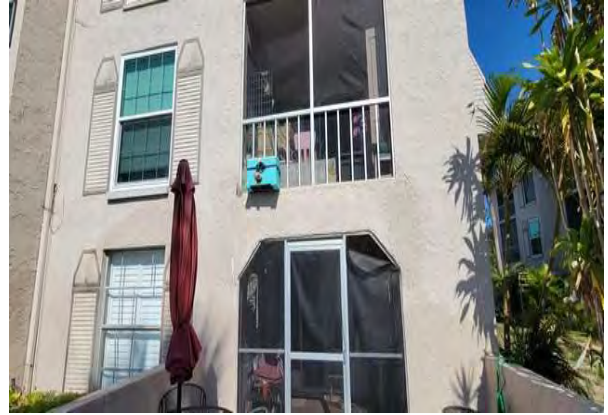
4 Left Rear Side of Building
