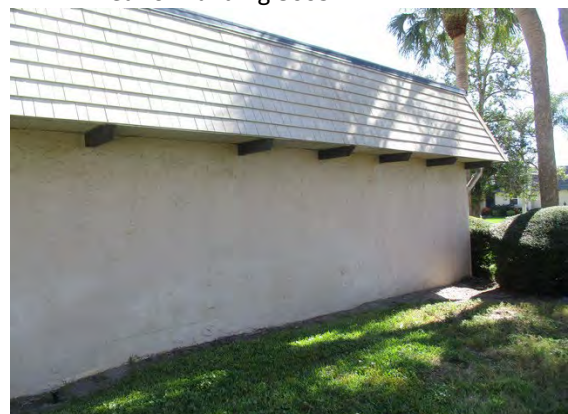
95 Left Side of Building 8605
