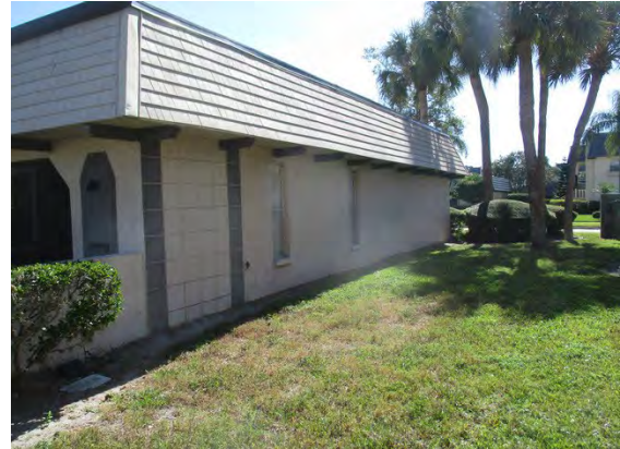
83 Left Side of Building 8605
