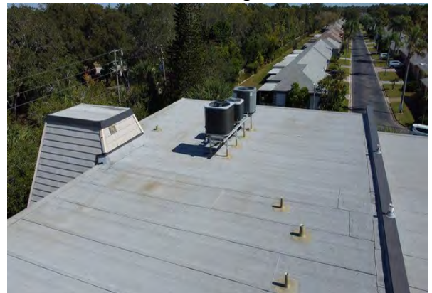
40 Roof Overview Building 8693
