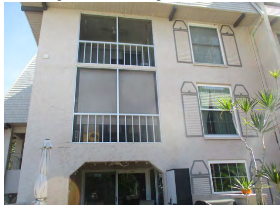
32 Rear of Building 8693
